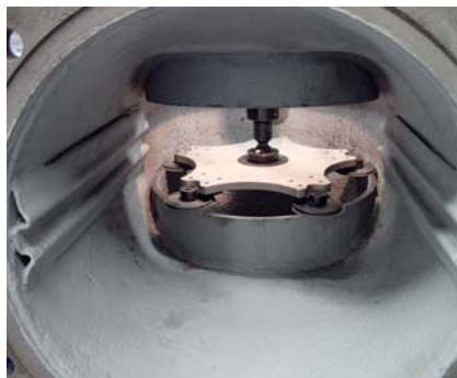
Grinding of gate valve
